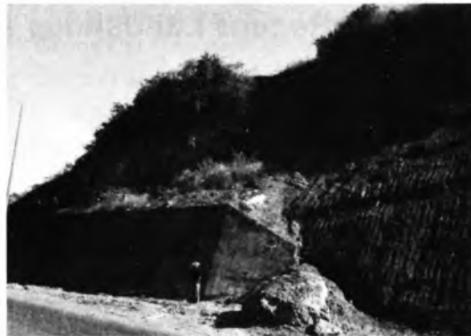
Photo 1. The debris slide on NH-4A Panjim-Ponda road. Retaining wall has to be extended.
