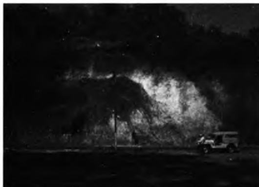
Photo 2: The debris slide at km 129 on NH-4A (Panjim- Ponda road).
